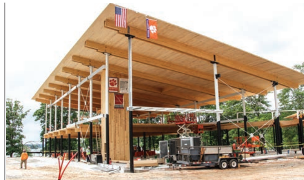
Clemson University's Snow Family Outdoor Fitness and Wellness Center is the first building made from southern pine cross laminated timber east of the Mississippi River.
